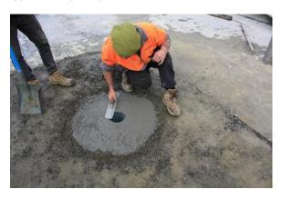
Note: If paving is to be placed over the top of the footing, the excavation must be deep enough to ensure that the concrete footing is minimum 40in/1000mm deep and 28in/700mm diameter.
