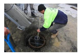
Fill the remainder of the hole with concrete. Ensuring that the application of concrete does not move the reo cage out of position.
